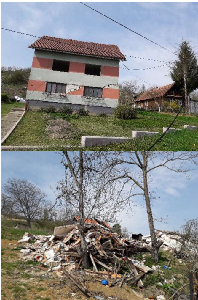
Figure 3 Houses destroyed by collapse of the Hrvatska Kostajnica landslide on 13 th March 2018.
